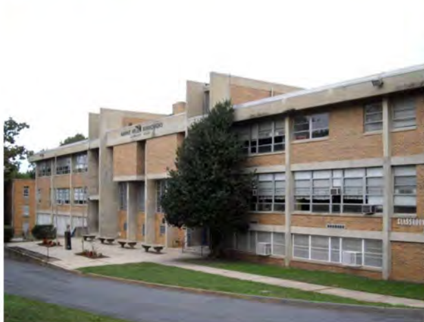
H School Building
